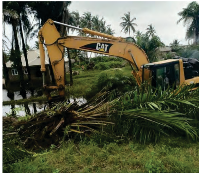
Tractor channelling and evacuating waterways in Lekki LCDA
